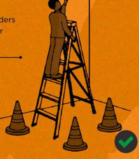
Do not work on the top rung of the ladder
